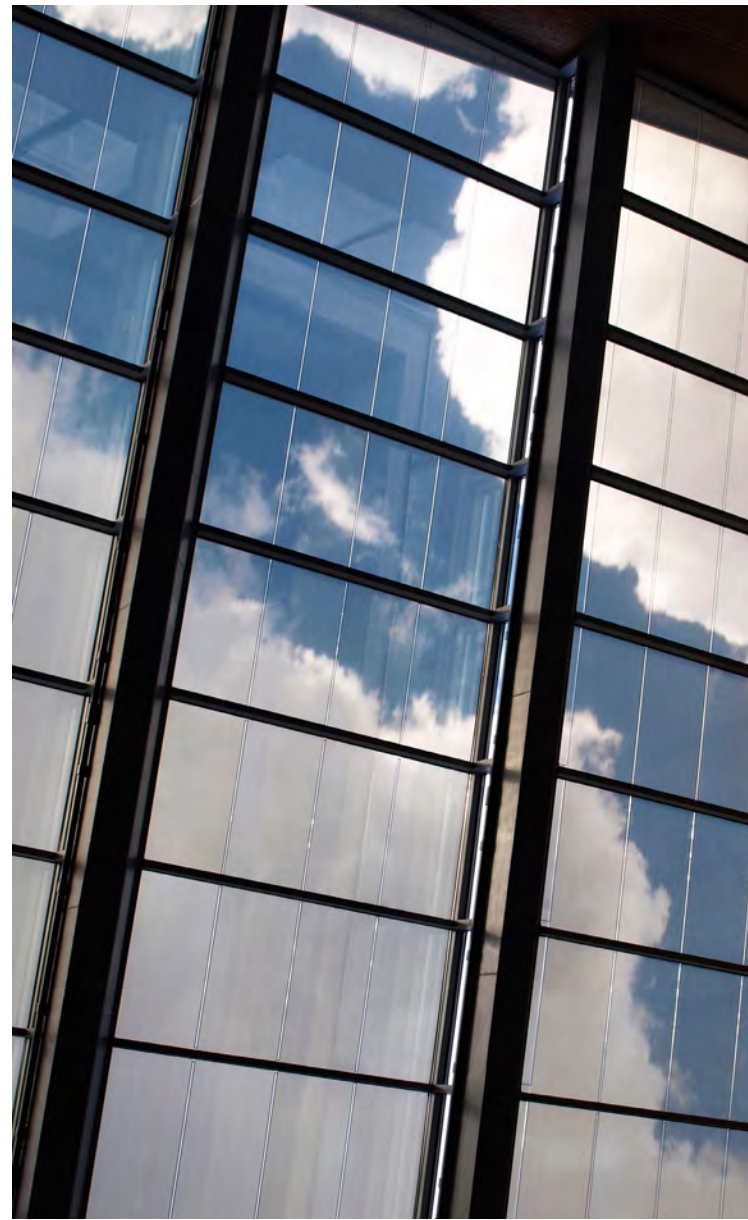
The pictures shown above belong to San Anton Market located in Madrid. This skylight is composed by photovoltaic glass with 20% of transparency degree.
