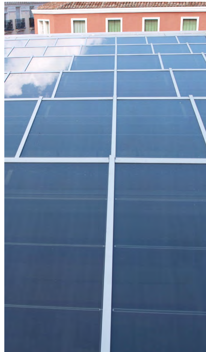
The pictures shown above belong to San Anton Market located in Madrid. This skylight is composed by photovoltaic glass with 20% of transparency degree.
